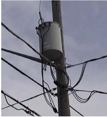
Photo A. Monophase transformer MV/LV
