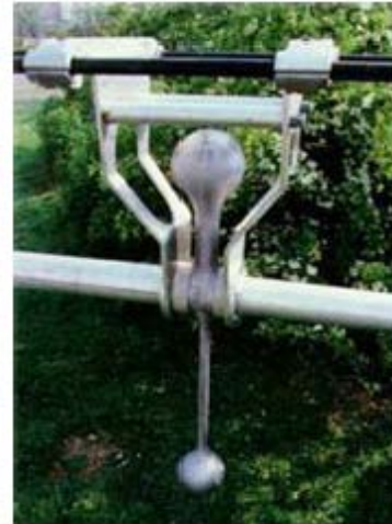
Fig.4. Photograph of The Torsional Damper and Detuner installed on the conductors (twin bundle)
