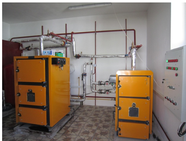
Briquettes fired boiler plant, Bilicenii Noi, Sangerei district
